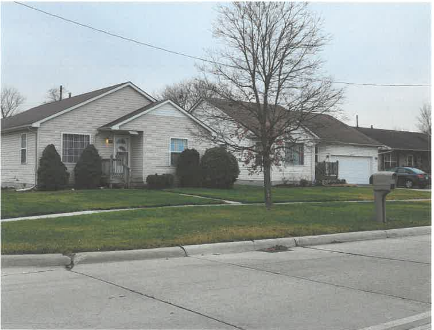
Annapolis Rd Infill Housing Westland
