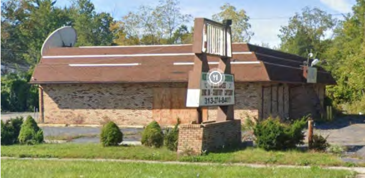
Figure 2 Existing building, eastern elevation
